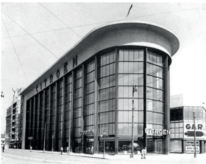
Showroom Citroën in Brussel. Archives d'Architecture Moderne (AAM), Brussel.
